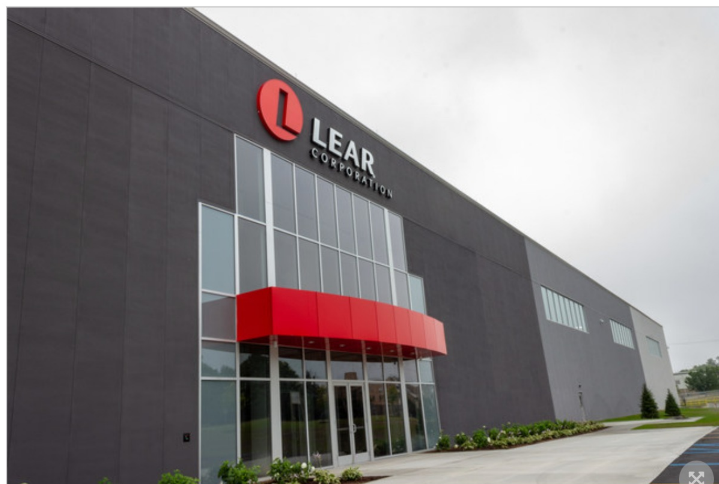
Lear Corporation Flint, MI Facility
